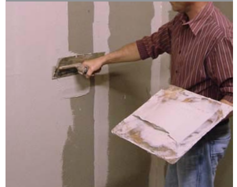
Plaster Skim Coat
