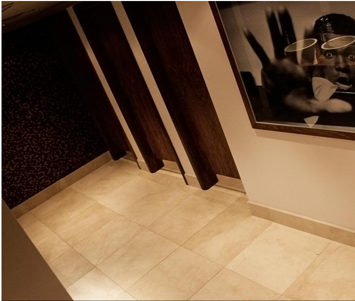
Custom cut skirting has been manufactured to match the tiling joints of the 60x60cm GOSS Apollo limestone tiles.
